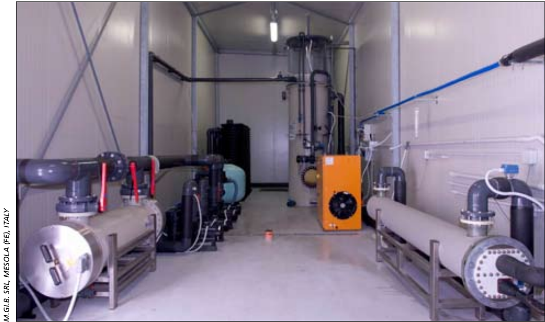
Figure 6.4: Two substantial UV units fitted in a large depuration plant
