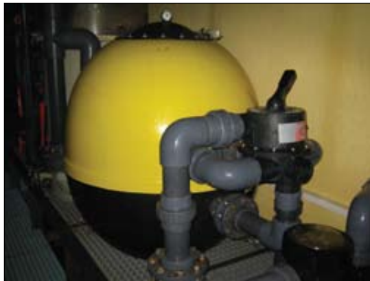
Figure 6.2: Pressurized sand filter used in a depuration system
